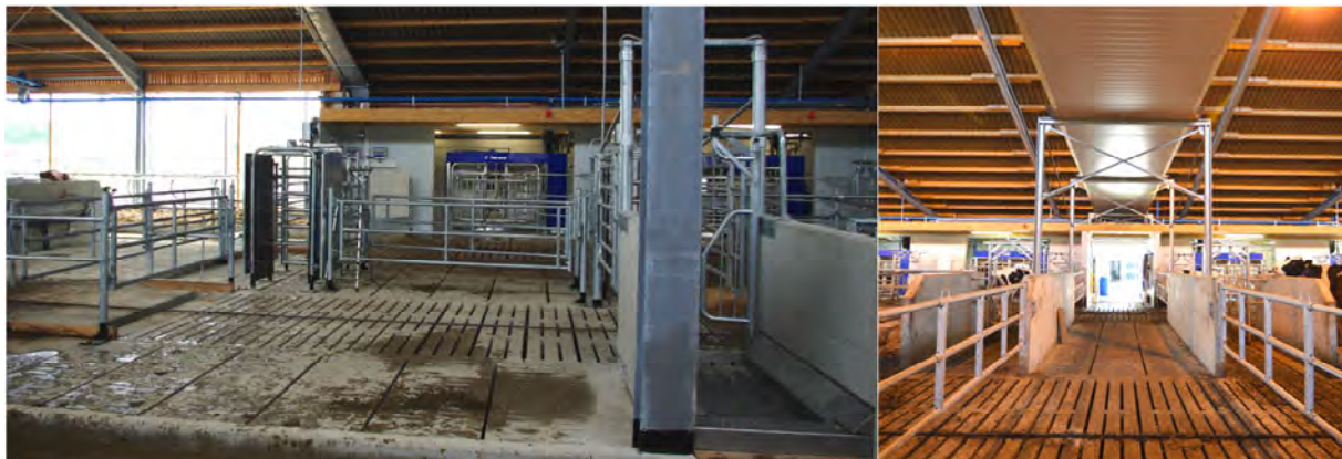
Figure 2: On the left picture is an AMS in the selection area and on the way out an automatic footbath, on the right picture is an inside view of the rooftop connection corridor
